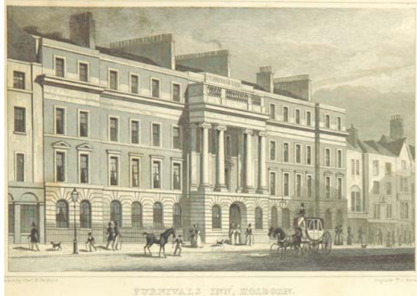
The three-storey Furnival's Inn, Holborn (1834-37)
